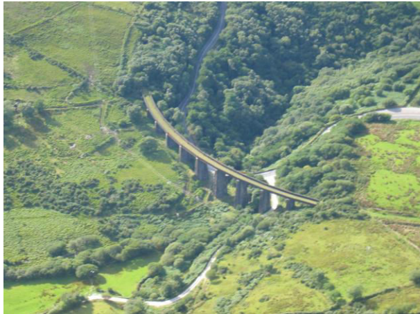
The Gleensk viaduct
